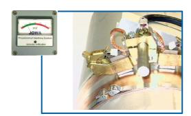
Constant contamination of silver surface increase the risk of spark erosion due to bad contact. Continous Slipring Cleaning Device prevents increase of the residual potential and keeps JOWA - PES in safe condition over long time.
